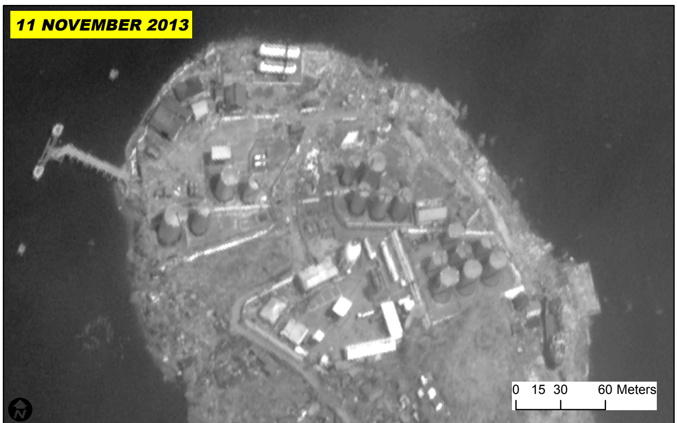
The Tacloban oil depot visibly intact in pre-crisis image (top) collected prior to Typhoon Haiyan. As of 11 November 2013 (bottom) many proximate structures and docks are eradicated with proximate debris indicative of complete destruction, and areas of tree cover are likewise destroyed. Primary depot buildings and tanks seem largely intact.
