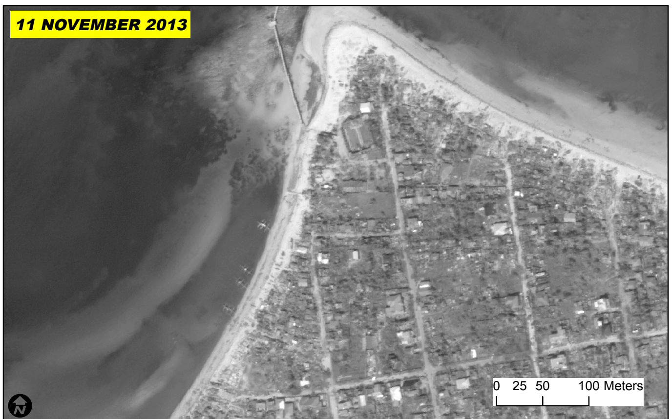
The northern end of the Madredijos municipality with multiple structures and tree cover visible intact in pre-crisis image (top) collected prior to Typhoon Haiyan. As of 11 November 2013 (bottom) most structures are gone with proximate debris indicative of complete destruction, and most tree cover likewise destroyed.
