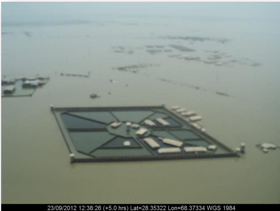
Picture 3: Photo of a large building on the route N-65 that has been severely flooded.
